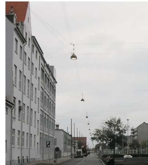
gatelys fra wire / streetlight mounted on wire
